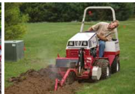
Light Footprint: Minimal Turf Damage & Work Mess
